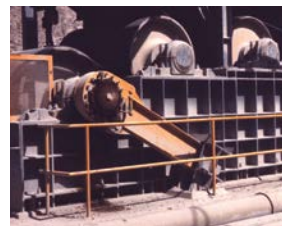
A Marland backstop installed on a large inclined mine conveyor prevents reverse rotation of the belt.
